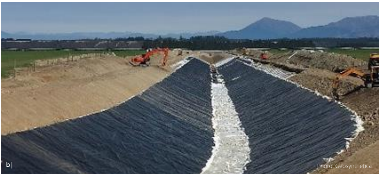
Figure 15 Canal linings a) concrete b) geotextile material
