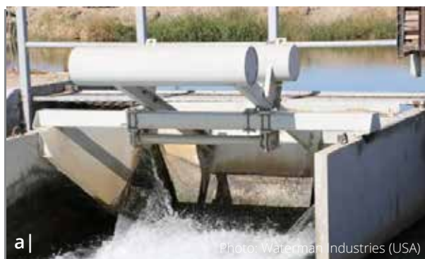
Figure 9 Automatic control of canal water levels a) Floating gate b) Duckbill weir
