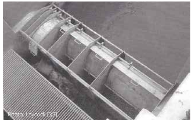
Figure 12 Baffle distributor that delivers a fixed discharge regardless of upstream water level. Variations in flow are made by opening different baffles.
