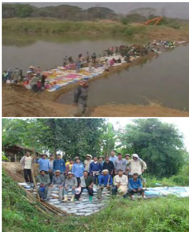
Figure 4.24 Water users group in Phrae province constructed a sandbag barrier to raise water level and pump to their farm lands
