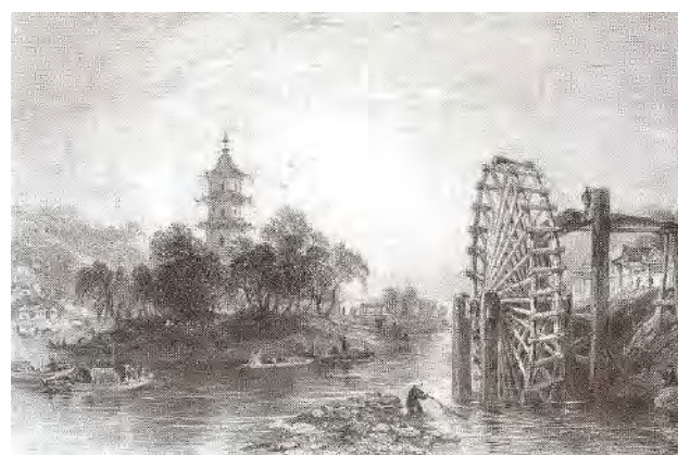
Figure 8. Hydraulic lifting water: the cylinder cars in working (drawn in the 19 th century). The diameter of cylinder car or water wheel is generally 2-3 m, which determines the height to lift water. Cylinder car was commonly used as urban and rural water utilities before the 20 th century
