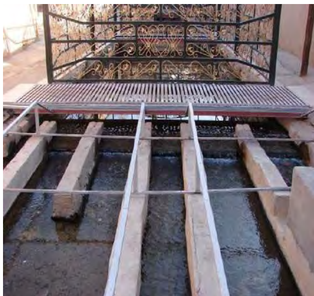
Figure 10. Maqdam; water dividing structure in the Qanat of Gowhar-riz, (Photo by Ali A. Semsar Yazdi)
