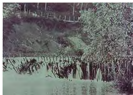
Figure 4. Wooden waterwheel and brushwood dam
