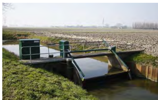
Figure 13. Weir controlling the upstream water level in a section of the Beemster
