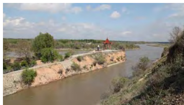
Figure 13. Diversion project of Yili River in Xinjiang: Chabuchaer canal headworks (built in the 17 th century, water diversion without dam)
