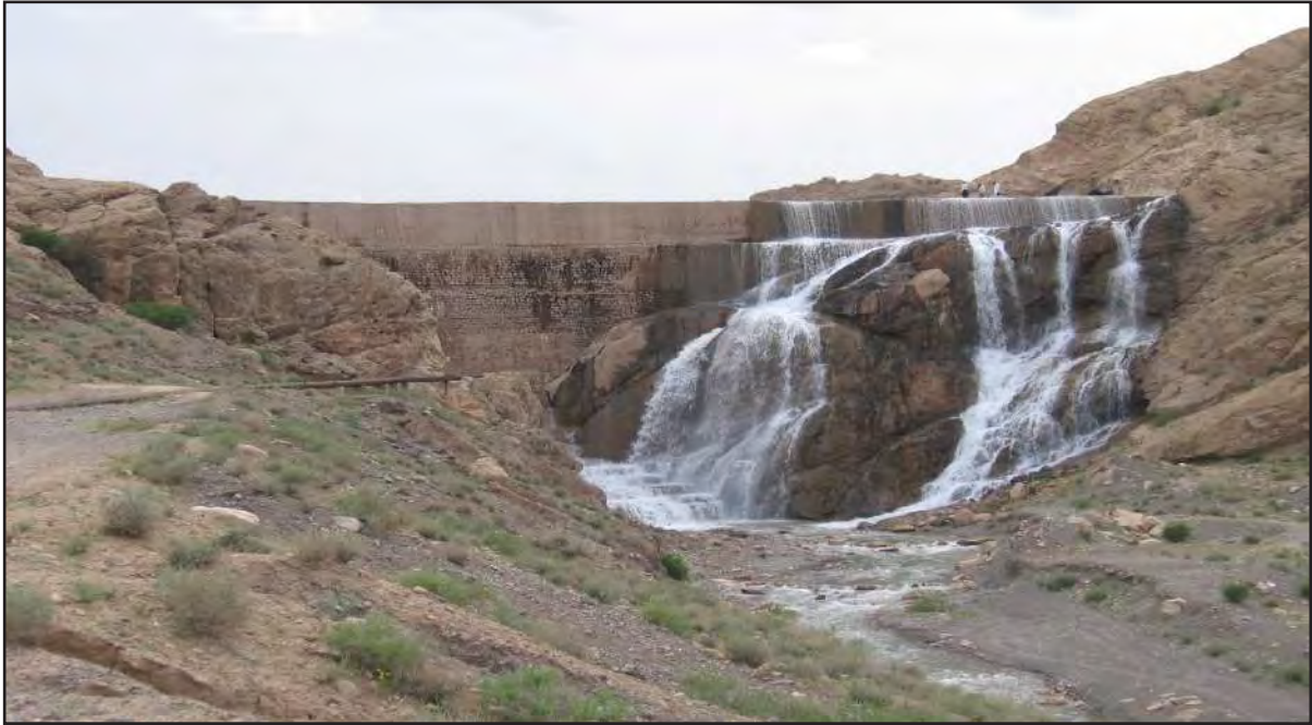
Figure 12. Historic dams: the 700-year-old Chebar dam, a combination of weight and arch dam, in Iran had a height of 22 m originally, the 3 m high concrete bar was added during rehabilitation work about 30 years ago
