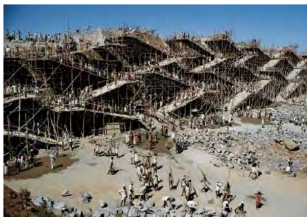
Figure 10: Workers swarm over scaffolding to erect the Nagarjuna Sagar dam, large masonry dam across Krishna River (National Geographic, May 1963)
