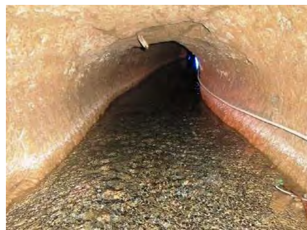
Figure 14. Xinjiang Karez (the junction section of culvert and open channel)
