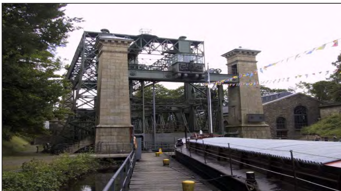
Figure 11. Old ship hoist at Henrichenburg (float lift), completed in 1899
