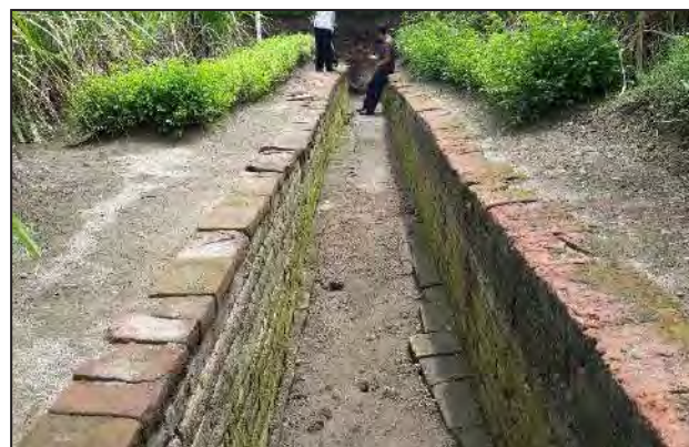
Figure 11. The ruin of irrigation channel made of brick layer with the size of 1.00 m x 1.00 m was excavated in Trowulan Village, East Java in 1990, estimated to be constructed during the Era of Majapahit Kingdom between the year of 1293 and 1500 (Gany, 3rd December 2014).
