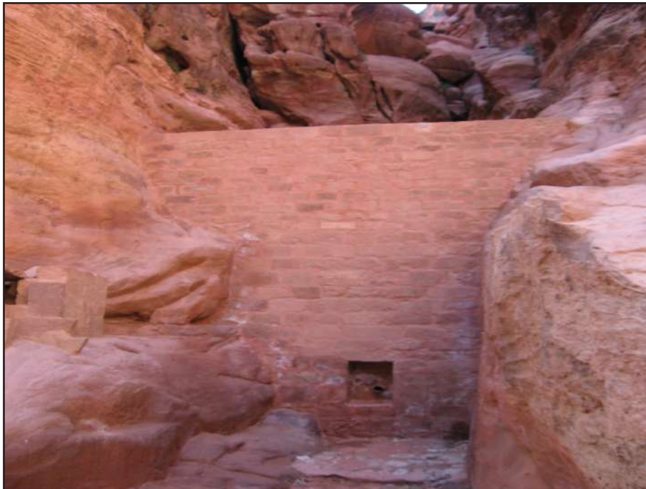
Figure 13. The flood protection wall modelled after the ancient original in the city of Petra, Jordan, with the wall keeping back flash floods in the neighbouring valleys
