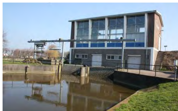
Figure 11. Electrical pumping station Jacobus Bouman on the Eastern side of the Beemster. One of the two fully automatic electrical drainage pumping stations
