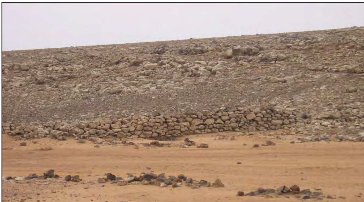
Figure 2. Ancient dams: remains of the dam at Jawa in the north-east of Jordan, one of the oldest dams in the world, originally standing about 5 m high
