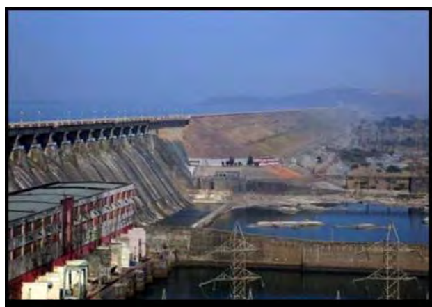
Figure 7 and 8: Hirakud Dam Project was the first Multipurpose Project in India. Completed in 1957, it provided irrigation to 2.51 lakh ha. Length of the dam (including dykes) is 25.5 Km (Water Resources Development in India, 1997, CWC)
