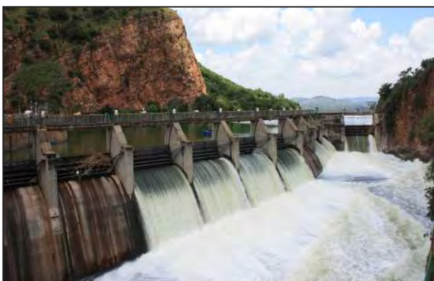
Figure 6. The Hartbeespoort Dam was originally completed in 1923 and raised through the addition of sluices (pictured) in 1970. (Lani van Vuuren personal collection)
