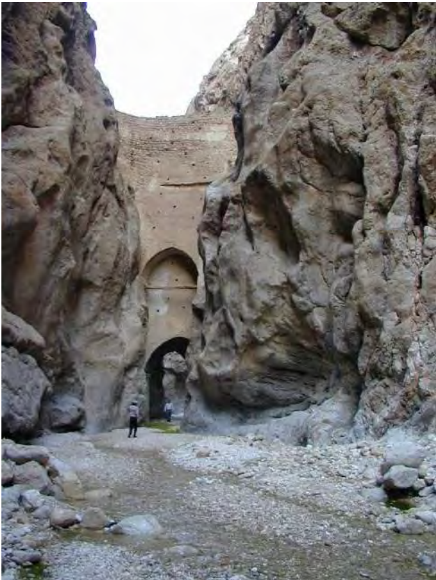
Figure 5. 25 m high Abbasi flood-retarding dam
