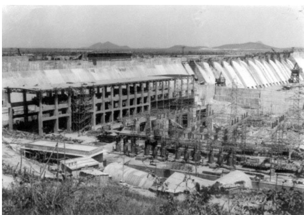
Figure 7 and 8: Hirakud Dam Project was the first Multipurpose Project in India. Completed in 1957, it provided irrigation to 2.51 lakh ha. Length of the dam (including dykes) is 25.5 Km (Water Resources Development in India, 1997, CWC)
