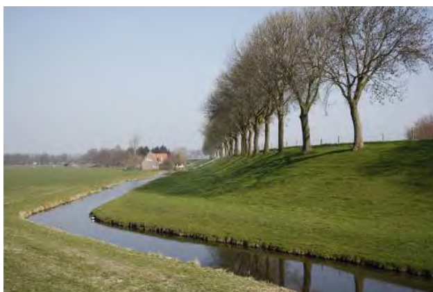
Figure 14. Inner side of the dike, with seepage drain, surrounding the Beemster
