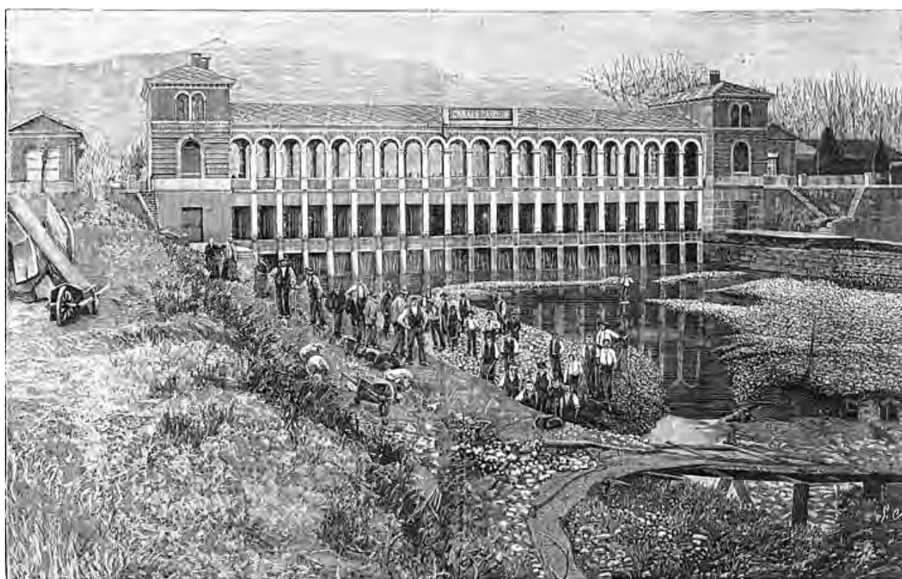
Figure 4. Entrance building of the waters of the Po into the Cavour Canal with the work almost complete (from a contemporary print)
