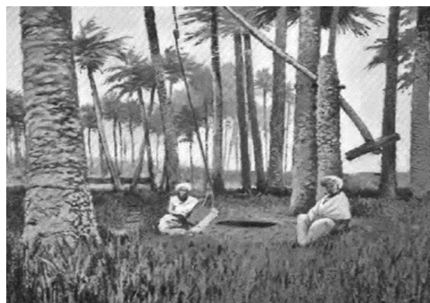
Figure 2: Paecottah or Lat was usually worked by two men for shallow lifts ('Irrigation in India' by Herbert M. Wilson, 2nd edition, USGS, 1903)
