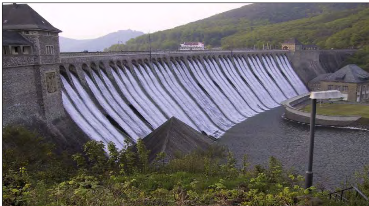
Figure 10. Edertal dam, gravity dam may of greywacke rubble, completed in 1914
