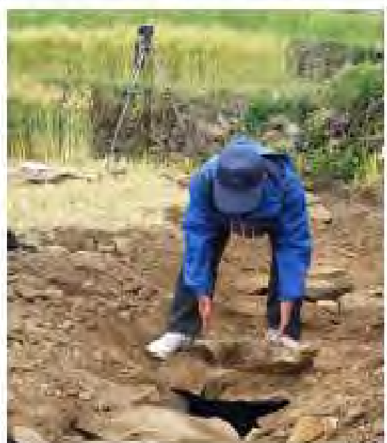
Repairing culvert cover with flat stone
