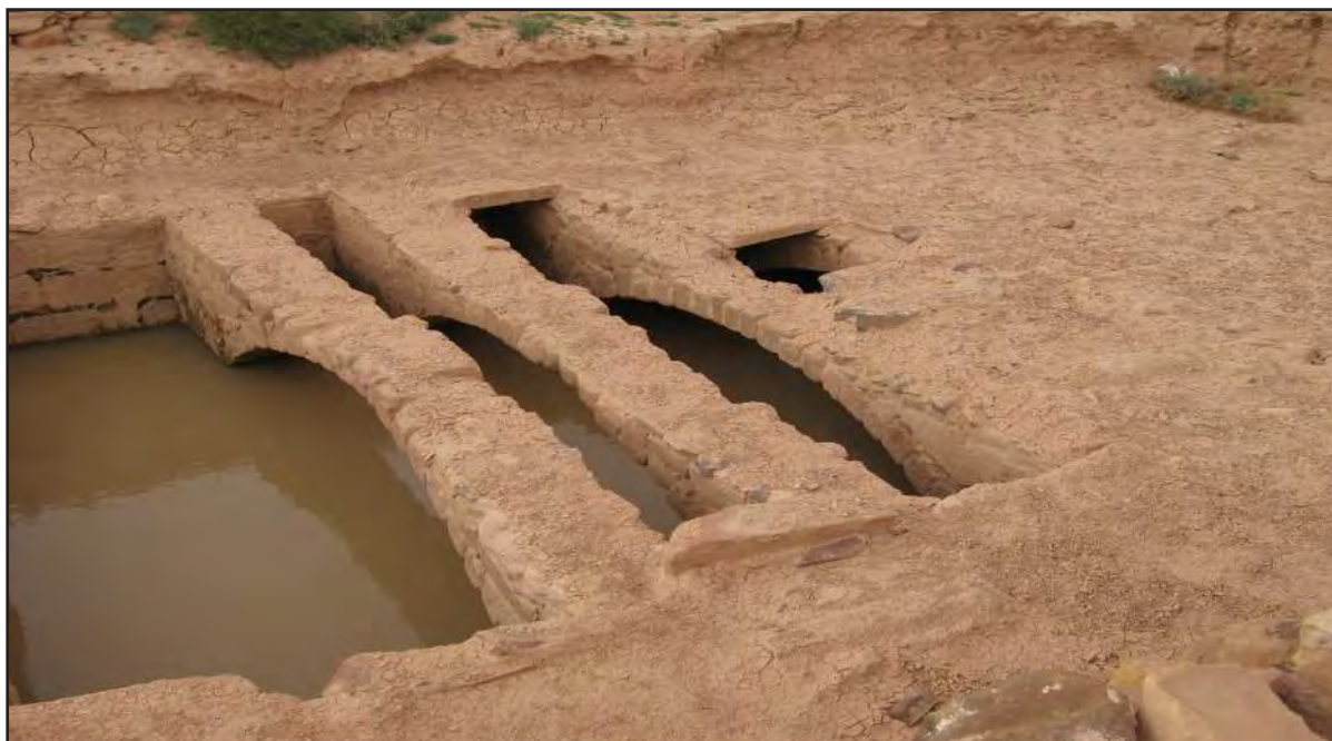
Figure 1. Large cistern for storing rainwater in the Nabatean city of Humayma
