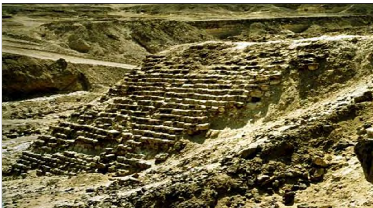
Figure 3. Sadd el-Kafara in Wadi Garawi, Egypt, 30 Km south of Cairo, height 14 m, a crest length of 113 m (right; photo: Henning Fahlbusch)
