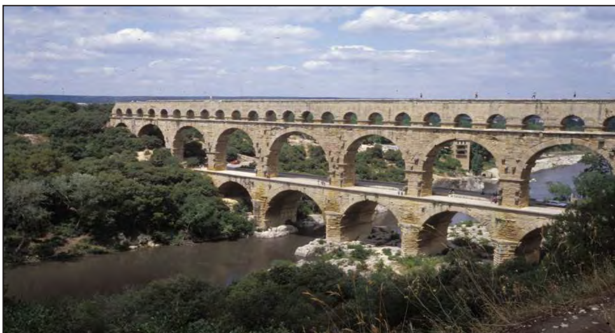
Figure 5. Pont du Gard along the 50 Km aqueduct of Nimes; the road bridge on the lower level was later erected over the aqueduct (right; photo: Henning Fahlbusch)
